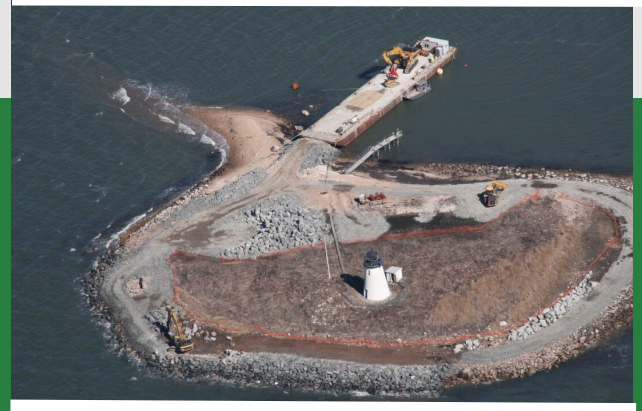
Drone photo of Bird Island during restoration. VIRIN: 160226-A-ME637-001.JPG
